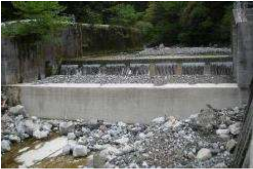
Stream Intake Works in normal time
