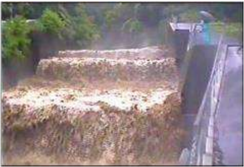
Stream intake works in flood time
